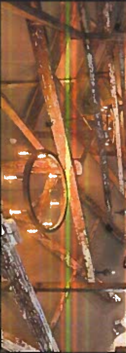
feature beams on first floor
